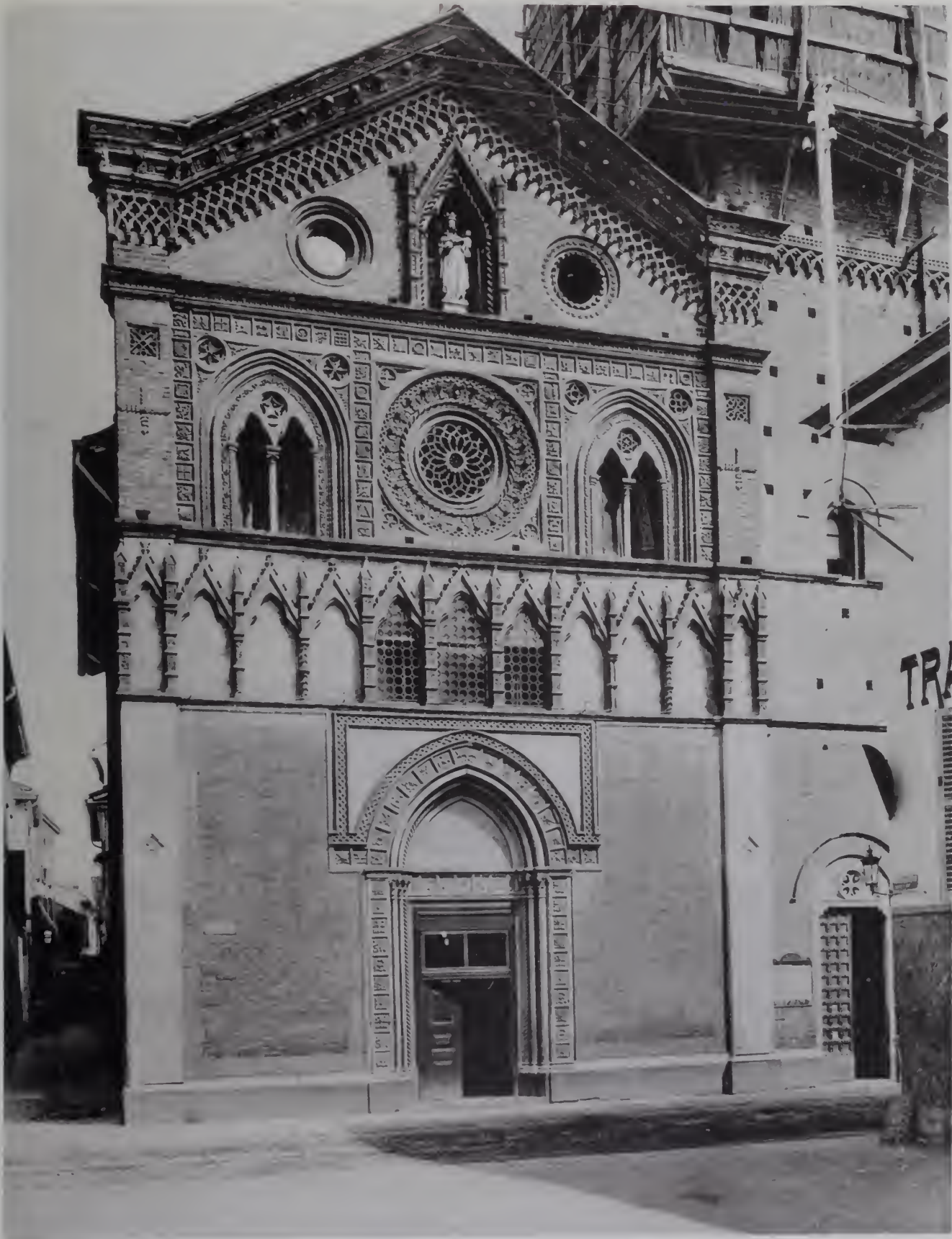
MONZA—CHURCH OF S. MARIA IN ISTRADA. REMARKABLE FOR ITS ELABORATE FRONT IN TERRA COTTA. 14TH CENTURY.
